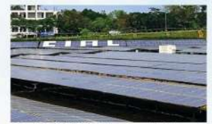
5.8 MWp Ground Mount Solar PV at CIAL
