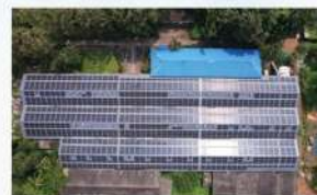
500 kWp Rooftop Solar PV at Traco Cable
