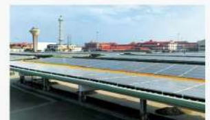
1.2 MWp Carport Solar PV at CIAL-Nedumbassery
